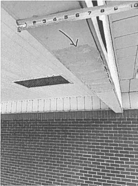
P-5 The underside of the steel beam has 6 1/2" approximate metal panel with that was damaged.
