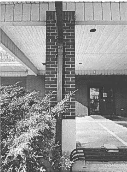
P-8 The brick pillars were in good-structural condition without any visible affects from the truck impact at the canopy roof.
