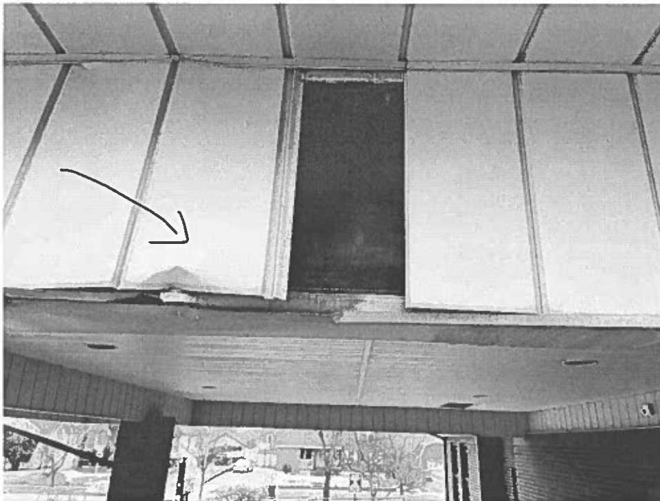
P-2 East Entrance canopy; Truck Impact Location at East Beam and Siding
