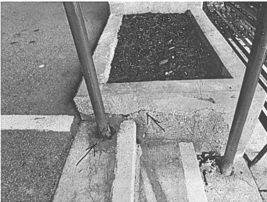
P-10 Planter curbs, Stairs & Railings. These have cracks and corrosion due to ag. Previous concrete repairs were made to the top of curbs. This area was not affected by truck impact to the carport Canopy-Overhang.
