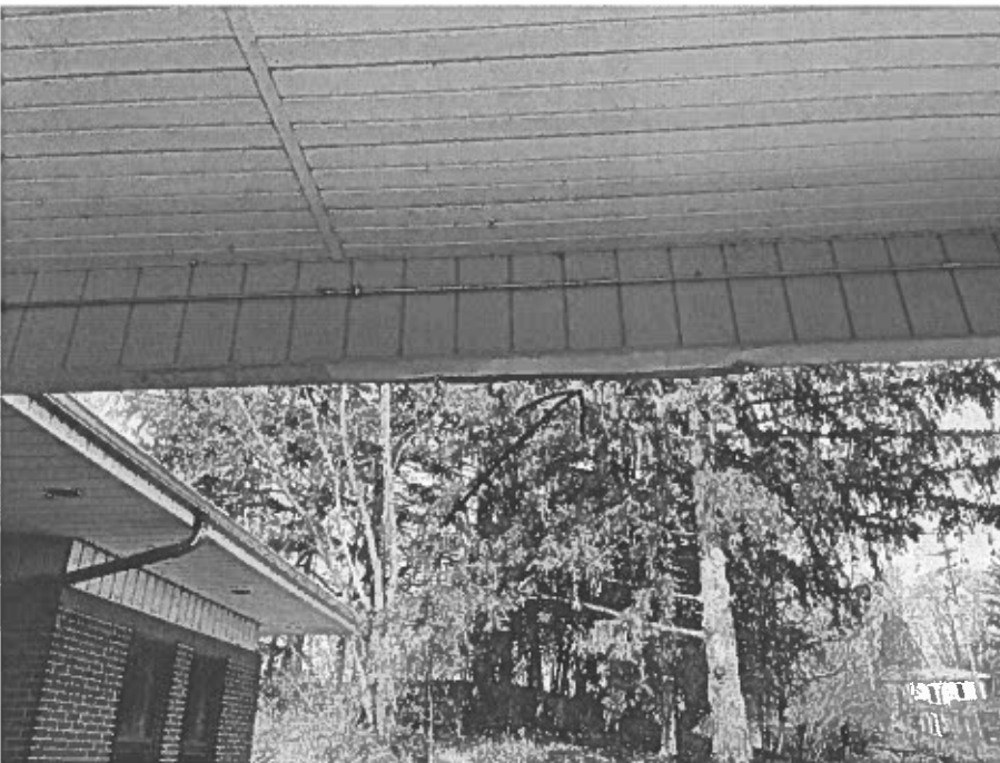
P-6 The far side and ceiling of the carport were undamaged. The bottom panel below the beam was bent and damaged as shown in Photo P-5
