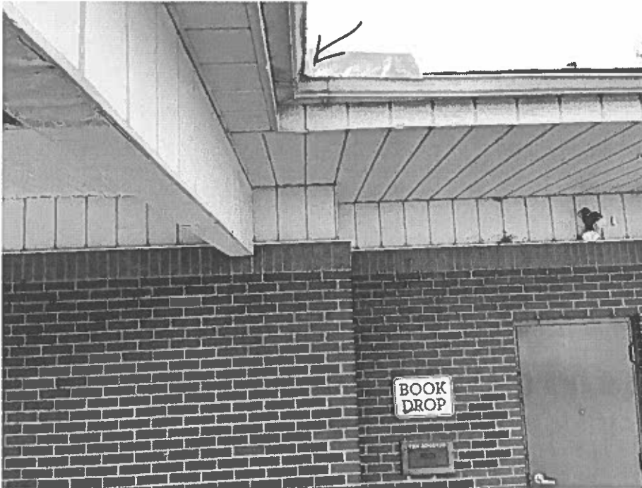
P-7 The gutters joining at the corner were affected by truck impact and baps joints and should be sealed with a gutter sealant.
